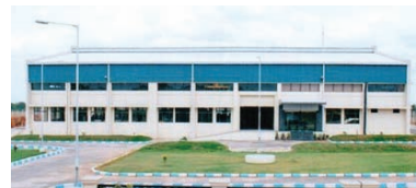
Pashamallaram Plant - Hyderabad: Power Transmission Accessories
