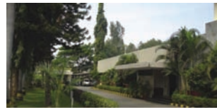
Patancheru Plant - Hyderabad : Belts, Oilseals and Moulded Rubber Products
